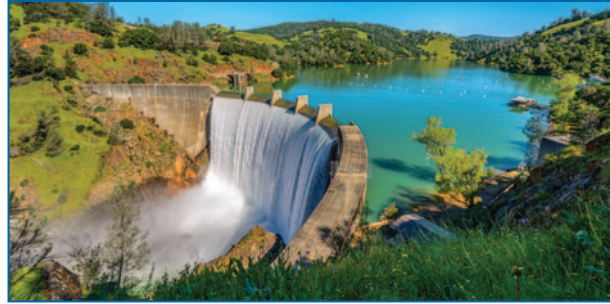
Englebright Dam on the Yuba River
